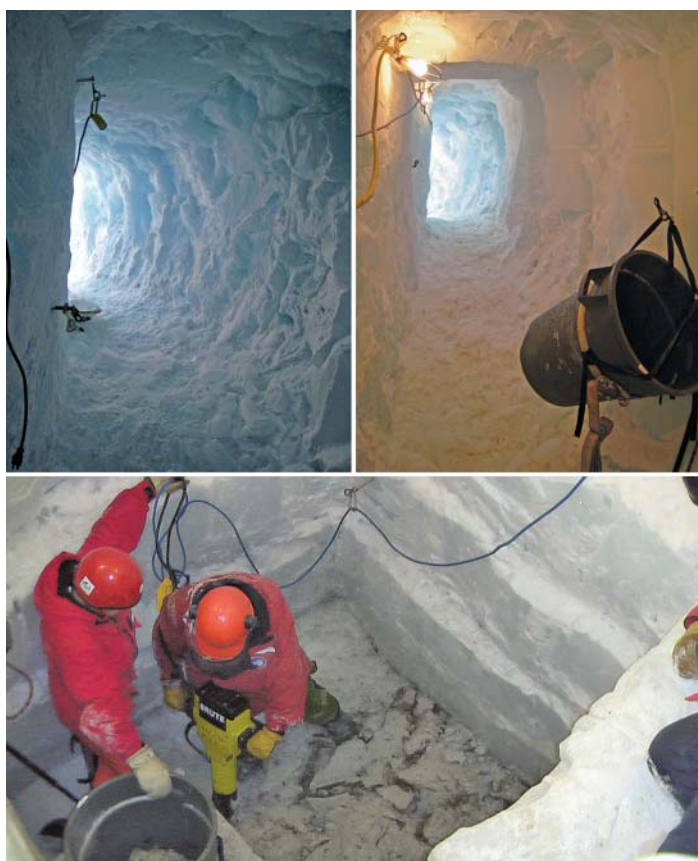
Fig 4, (upper left) Up-sloping initial 4 m of tunnel. Fig 5, (upper right) down-sloping 9 m portion of the tunnel. Fig 6, (bottom) 5 m shaft being dug.
